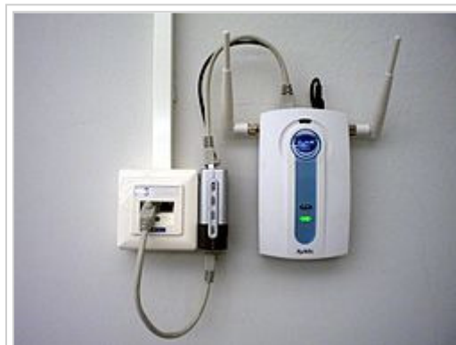
Wireless LAN access point, powered by a PoE splitter
